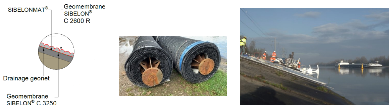
Figure 6. Kembs. Cross section of the Sibelonmat®, rolled void mattresses ready for installation (the drainage geonet is the black material, and the integrated zips is visible along the edge of the mattresses), and the Sibelonmat® deployed on the slope with navigation ongoing during underwater works.
