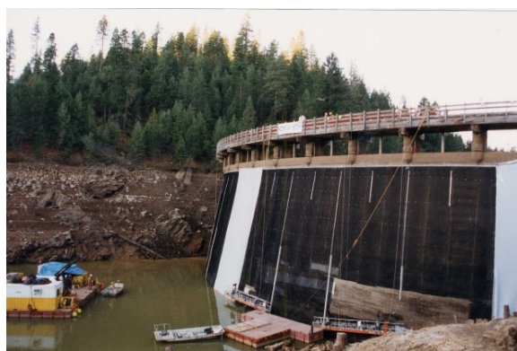
Figure 1. Lost Creek. At left, the grey geocomposite sheet under placement over the black drainage geonet, and the first components of the vertical anchorage assembly. At right, the anchorage profiles waterproofed in the dry section. The closer spacing of profiles in the top area can be seen.
