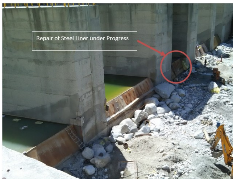
Figure 4. Steel liner at the end of roller bucket
