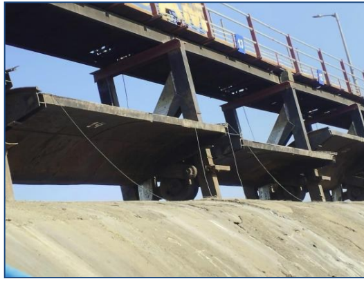
Fig 1. Excessive Corrosion in 2023
