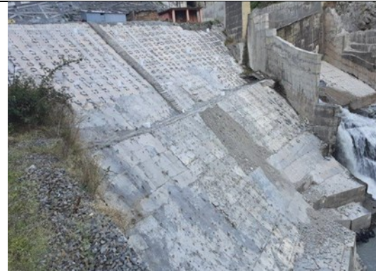
Restoration of D/s slope after repair
