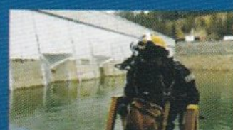
Buttress dam, underwater rehabilitation Exposed Sibelon® geomembrane Studena, Bulgaria (ongoing)
