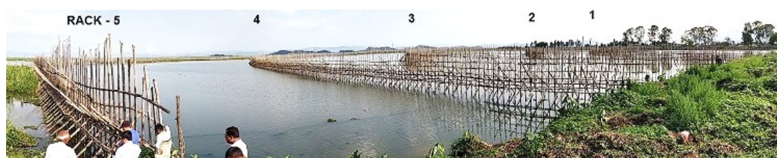
Figure-5: View of the Bamboo trash rack at Power channel
