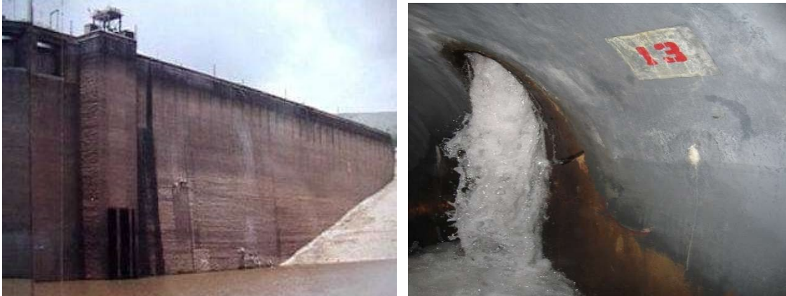
Figure 1&2 Condition of the Kadamparai Dam before Geomembrane Installation
