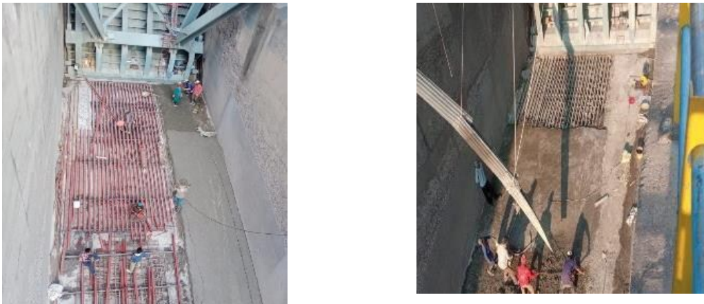
Figure 13. Placement of M80S grade concrete on the right side of the existing rails.
