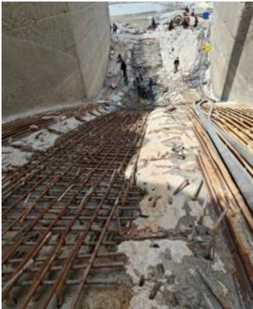
Figure 11. Surface preparation and laying of reinforcement of sluice spillway at Radial Gate No. 4.
