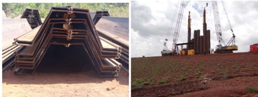
Photo 1. Paired sheet piles delivered on the jobsite (left), driving on the dam crest (right)
