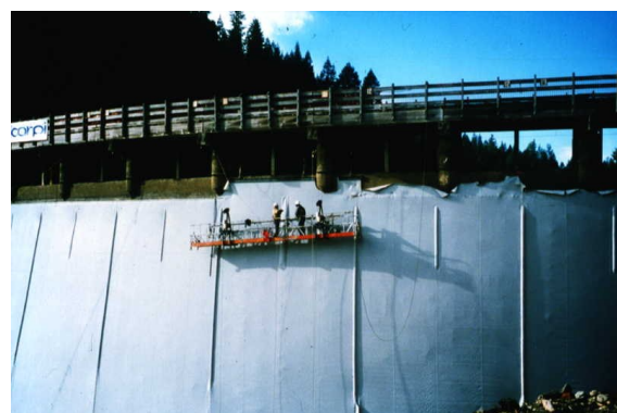
Figure 1. Lost Creek. At left, the grey geocomposite sheet under placement over the black drainage geonet, and the first components of the vertical anchorage assembly. At right, the anchorage profiles waterproofed in the dry section. The closer spacing of profiles in the top area can be seen.
