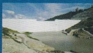
RCC dam, new construction Exposed Sibelon® geomembrane Susu, Malaysia
