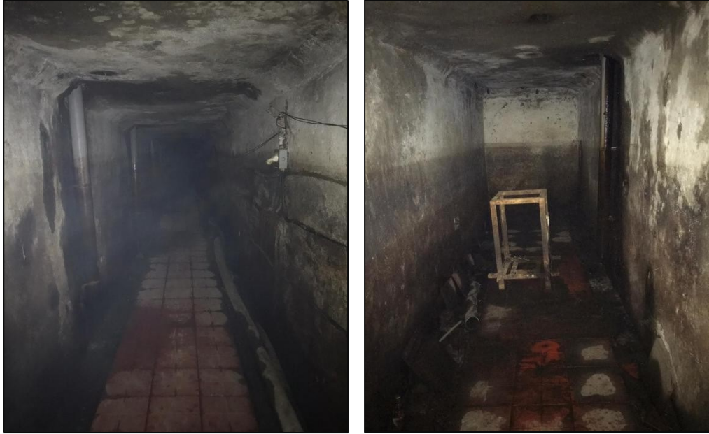
Figure 4 Observation of dryness in inspection gallery in 2016 - Totally dry
