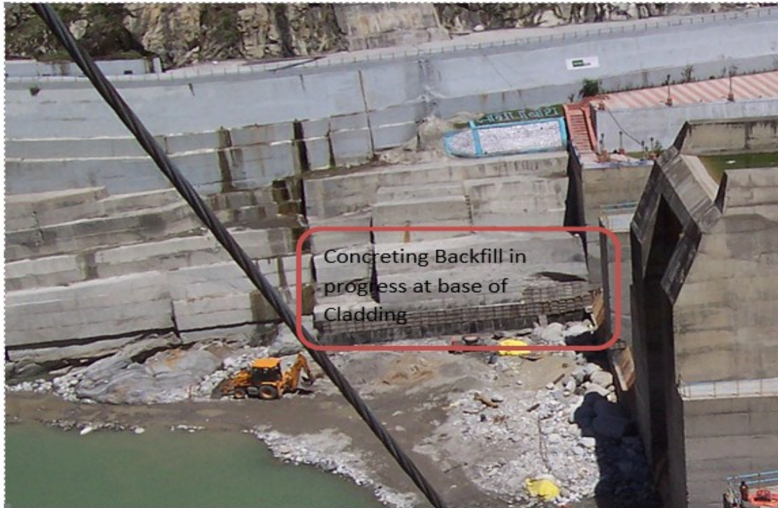
Figure 5. Concreting Backfill in progress at base of Cladding.
