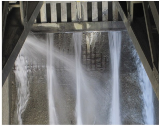
Erosion in Spillway Glacis
