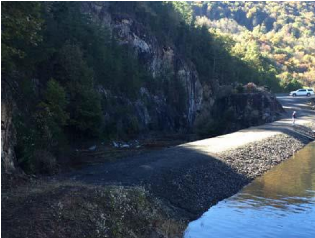
Figure 3 Auxiliary spillway with fuse plug
