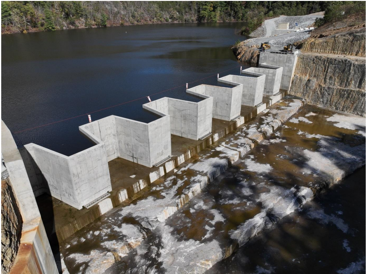
Figure 15 Fusegates downstream view in operation
