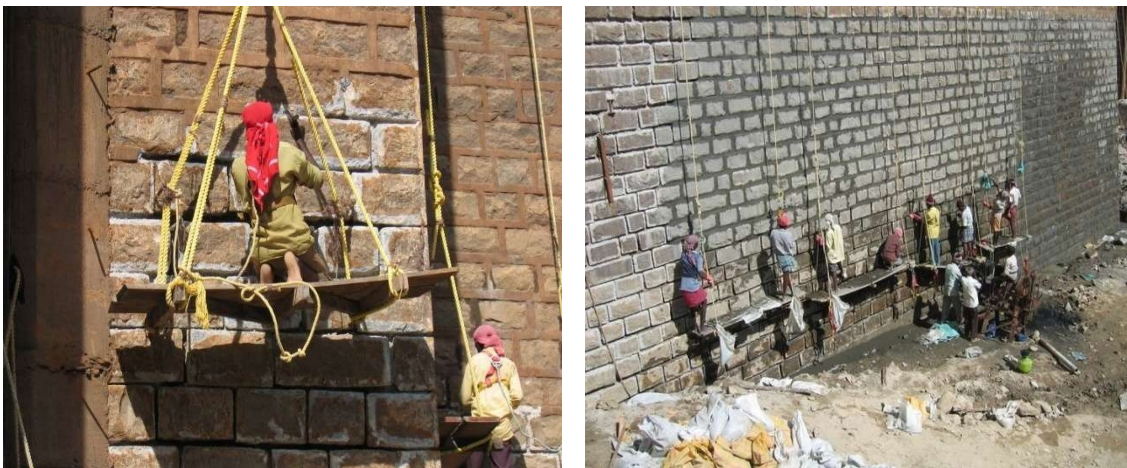
Figure 3&4 Conventional Racking and packing treatment methods carried out
