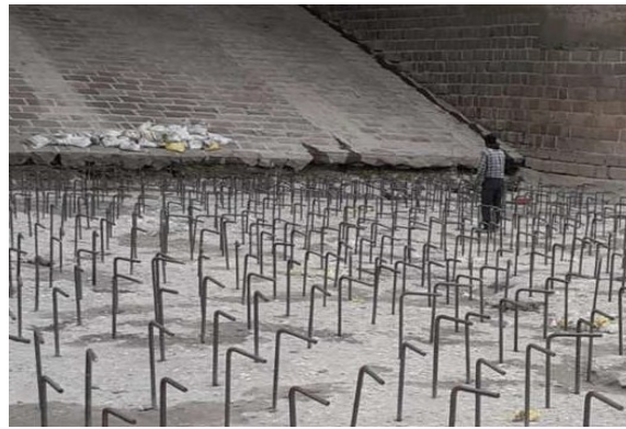
Figure 4. Ongoing repair work in stilling basin area
