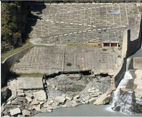
Erosion of D/s slope before repair
