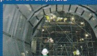
Pressure tunnel, rehabilitation Exposed Sibelon® geomembrane Helms, USA
