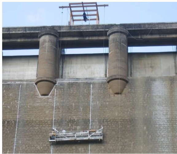
Figure 6 Laying of Vertical anchorage lines minimum reinforcement
