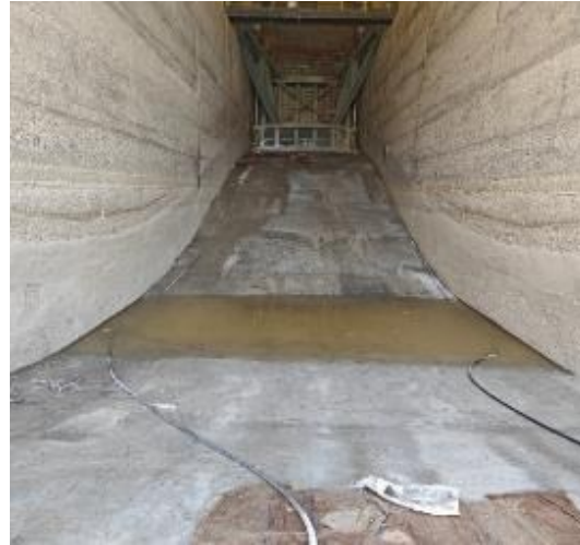
Figure 10. Repaired sluice spillway at Radial Gate No. 3.
