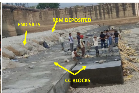
Figure 6. Repair of Launching apron with CC blocks
