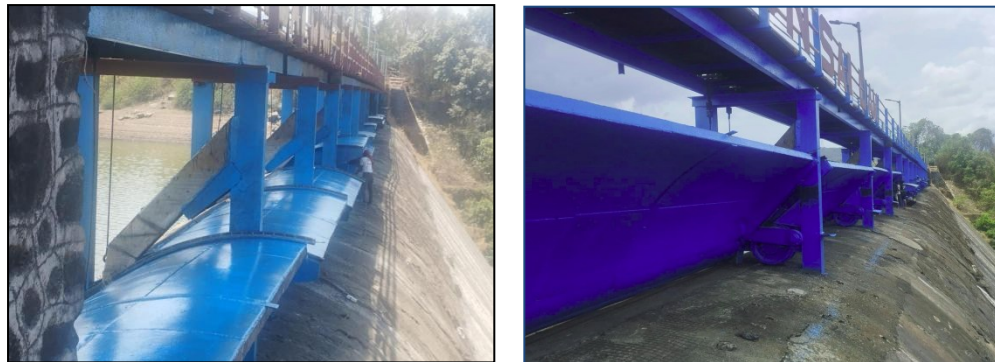
Figure 4. After Completion of Corrosion Protection Work of All Gates
