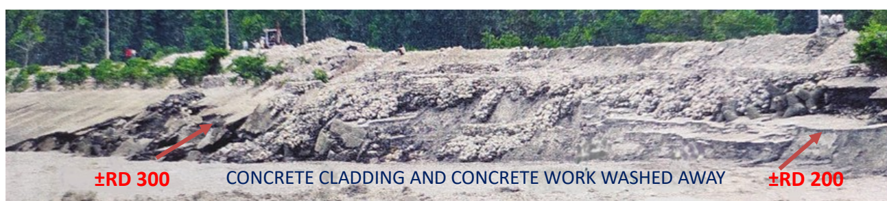
Figure 3. View of damages in Left afflux bund after monsoon 2013 flood
