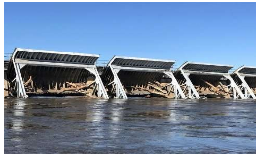
Figure 5: Debris stuck in dam gate
