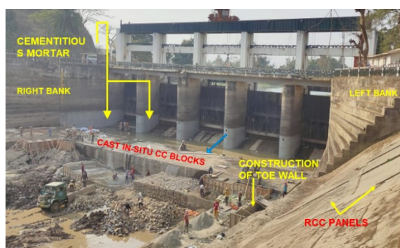
Figure-3:- Ongoing repair work in stilling basin
