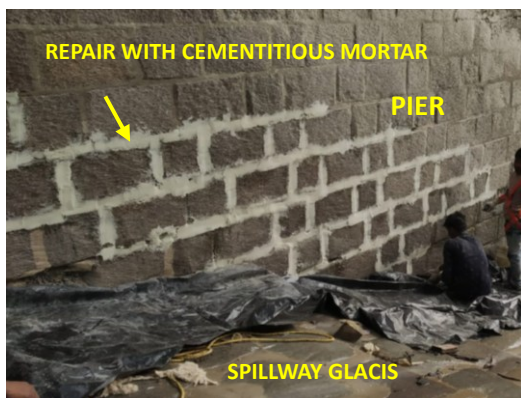
Figure 5. Repair work in Spillway pier
