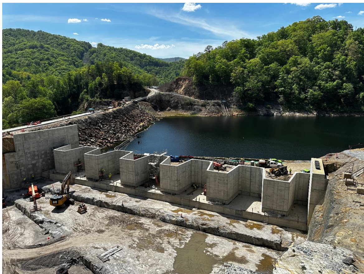
Figure 14 Fusegates downstream view after completion (during the as built survey)
