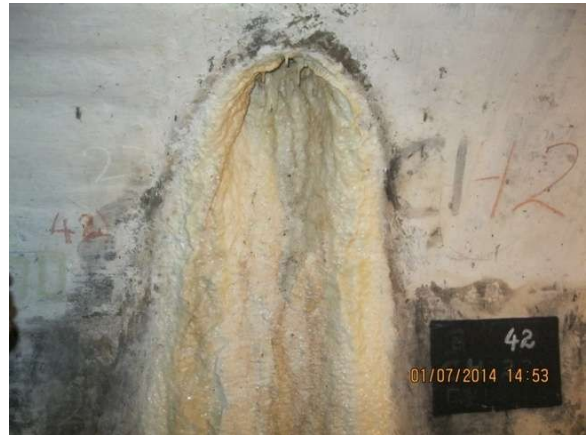
Fig 12. Choked Drainage Shaft
