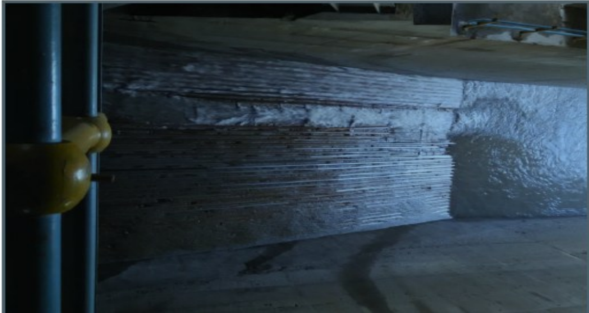
Figure 6. Damaged floor of under sluice
