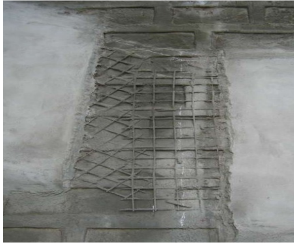
Figure 5 Surface Preparation by Shotcreting with minimum reinforcement
