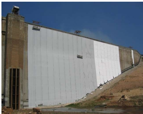
Figure 7 Placement of Geocomposite over Geotextile layer
