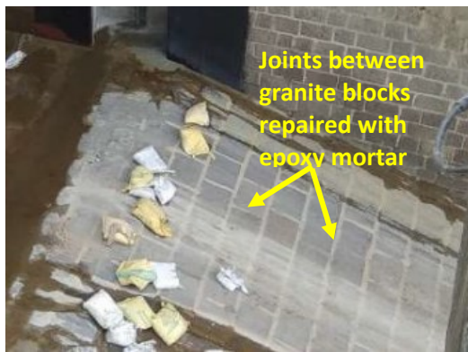
Figure 3. Repair done in spillway glacis
