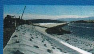
Hydropower canal, rehabilitation Sibelon® geomembrane partially ballasted Tekapo, New Zealand
