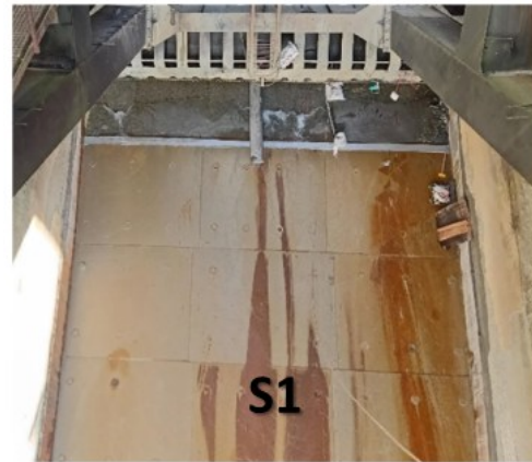
Restoration of Glacis with steel liner
